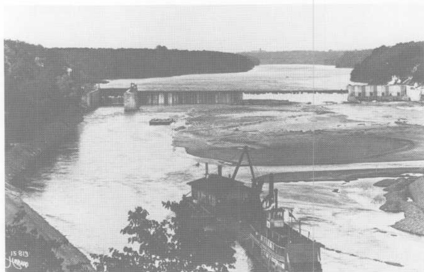
Twin City Lock and Dam No. 1, also known as Lock and Dam No. 1, the “high” dam, or the Ford dam, is located six miles below the Falls of St. Anthony. In the late 1920s, sewage and industrial wastes from both Minneapolis and St. Paul collected in the river above the dam.
