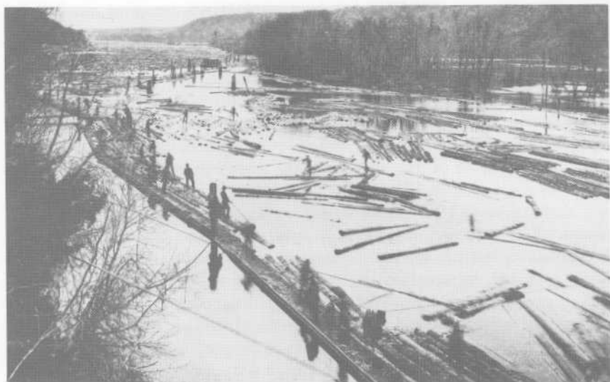
Logs were collected at boom sites to be arranged into huge rafts for further transport. This is the St. Croix boom in 1886.
