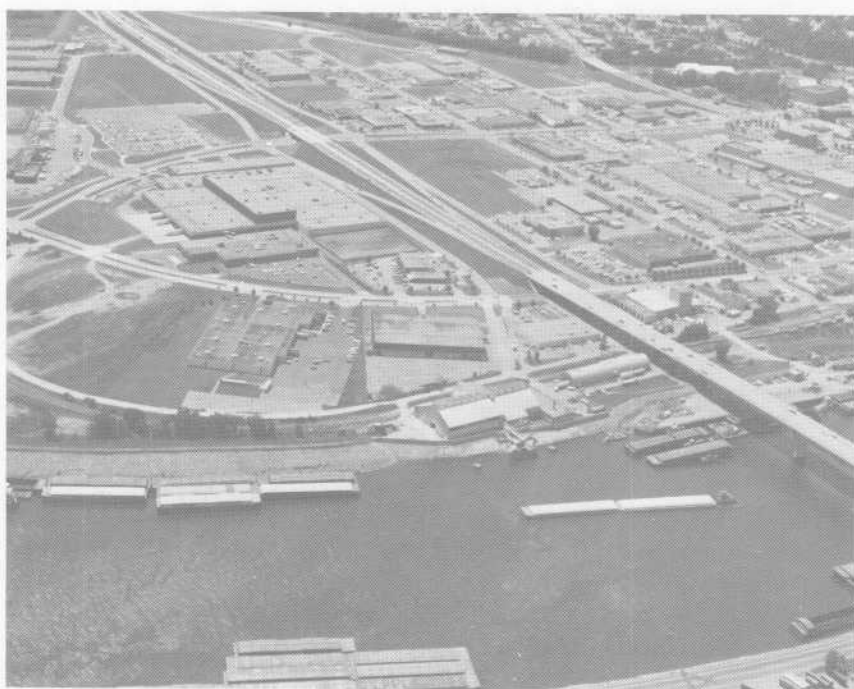
The St. Paul industrial floodplain in 1981. The "new" bridge is at far right. The levees and floodwalls are visible along the river.
